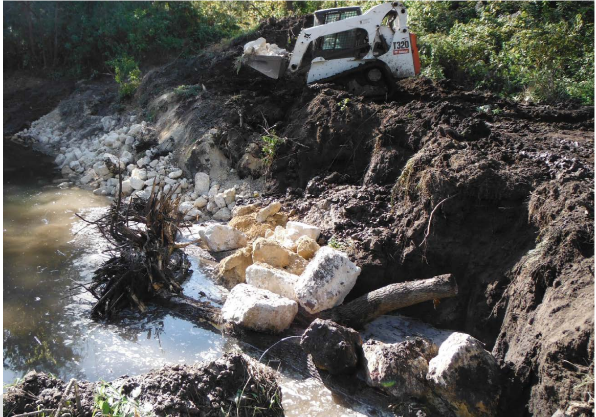
Figure 8: Rootwad Placement (Haring).
