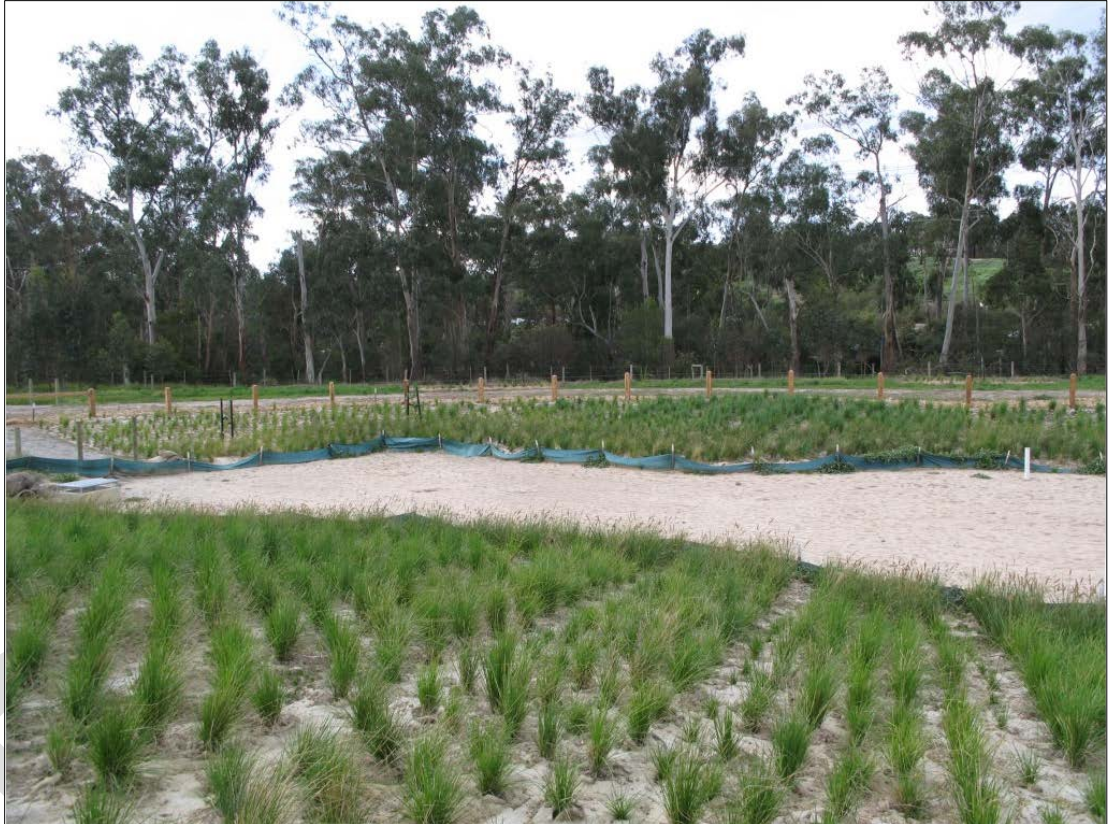
Figure 18: Created Wetland under Construction (Wikimedia Commons)
