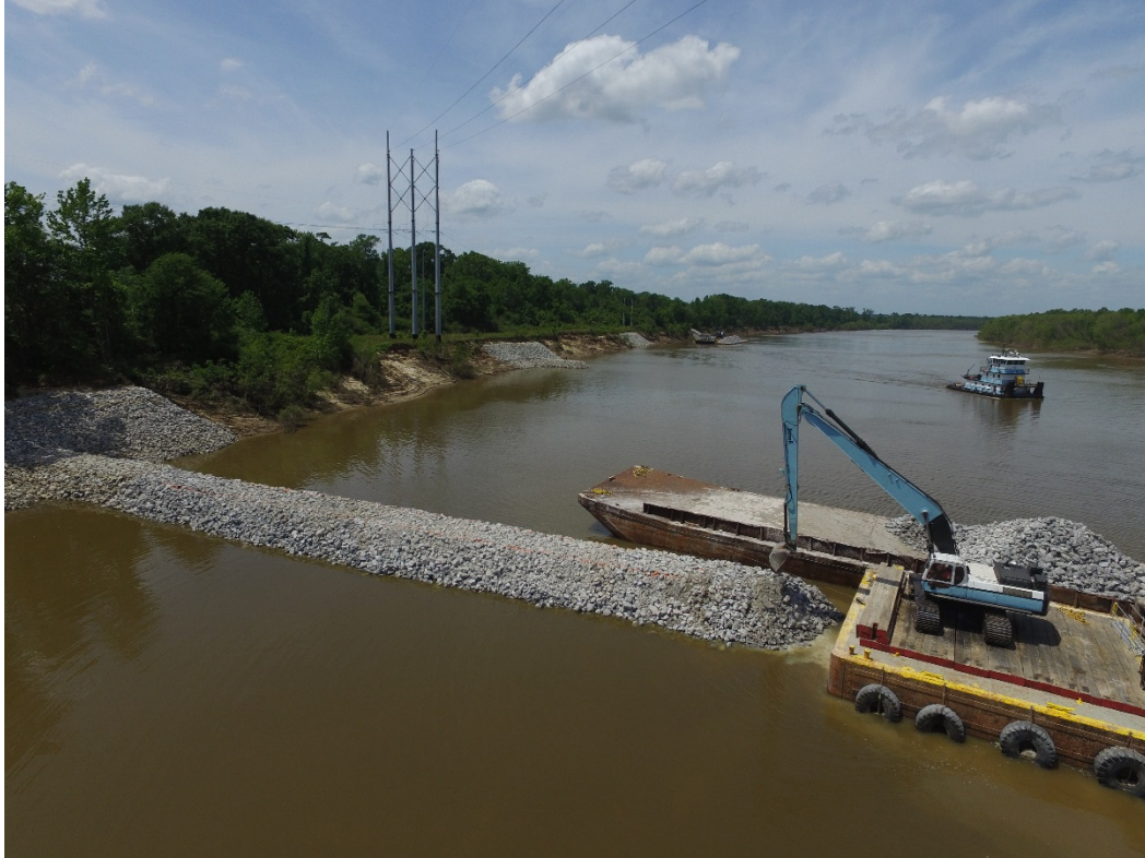
Figure 13: Construction of Training Dikes.
