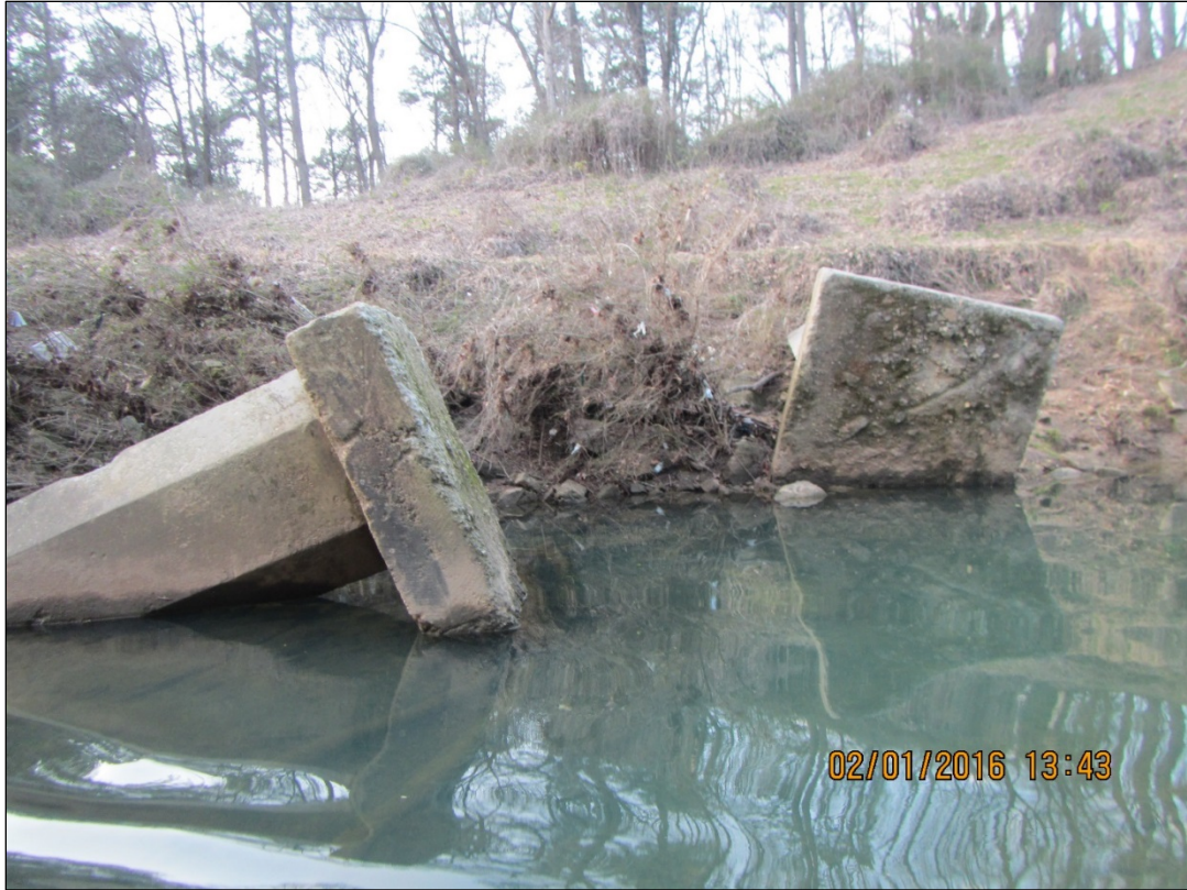
Figure 17: In-situ concrete piers near PC-08
