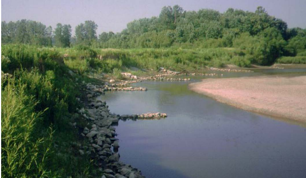
Figure 12: Bendway Weirs. (Haring)
